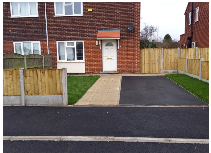
Vico Homes Environmental scheme approved driveway (drainage channel to front).
